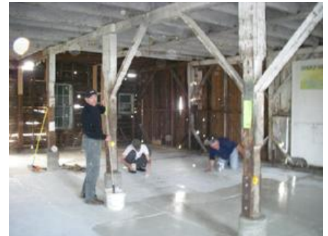
Priming and painting the new floor
