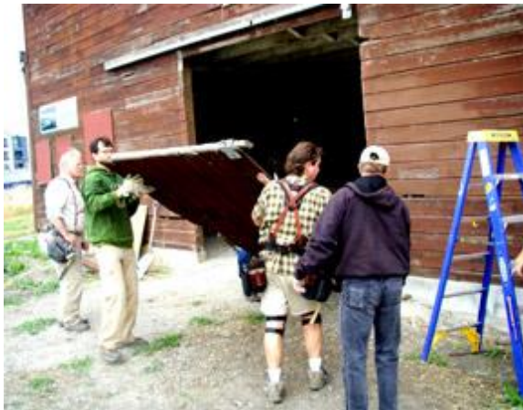
Team Torch builds new doors for the Livery Stable
