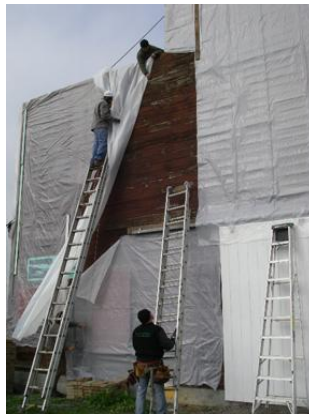
Placing plastic on the façade
